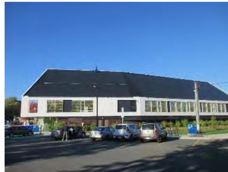
Photo showing PV systems and south facade
