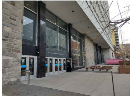
V6 - View of Rue Bishop entrance looking towards Rue Sherbrooke O.
