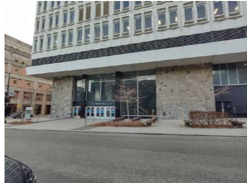
V7 - Rue Bishop exterior facade looking towards Boul. de Maisonneuve O.
