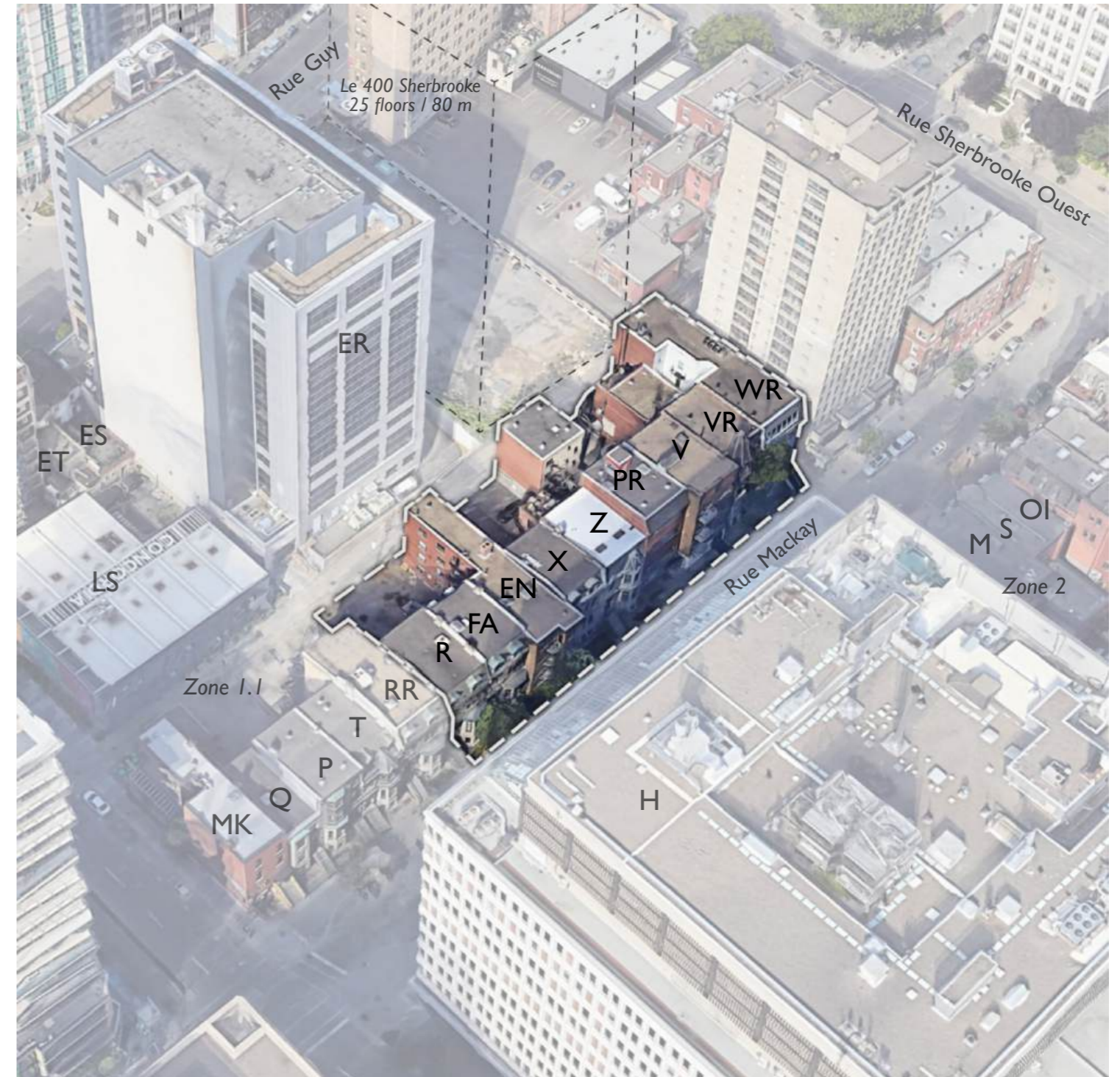
Aerial view of existing conditions
