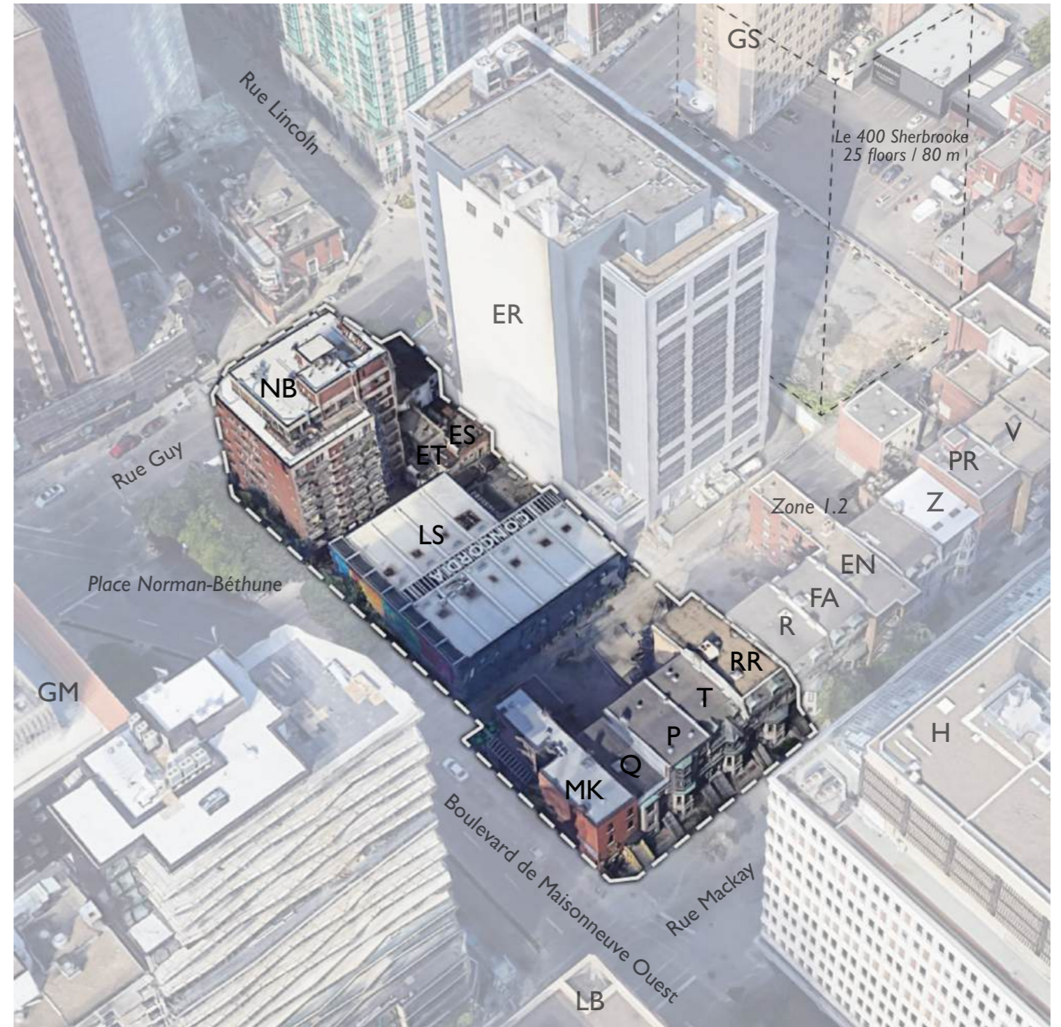
Aerial view of existing conditions
