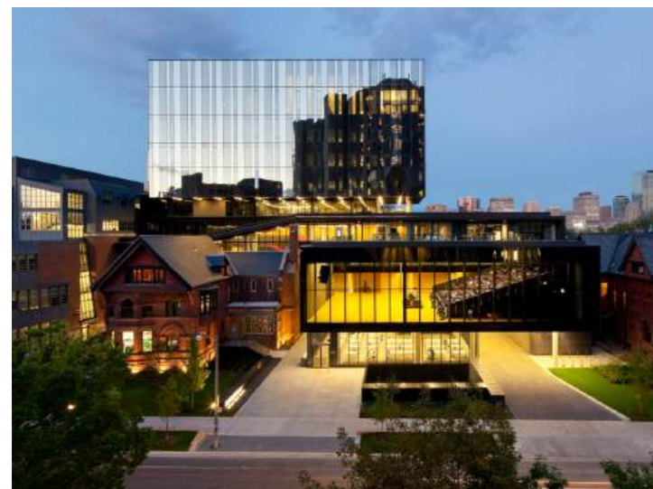
The Joseph L. Rotman School of Management Expansion Toronto, Canada – KPMB Architects, Tom Arban
