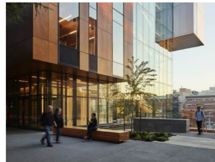
Life Sciences Building, University of Washington Washington, United States – Perkins+Will, Kevin Scott
