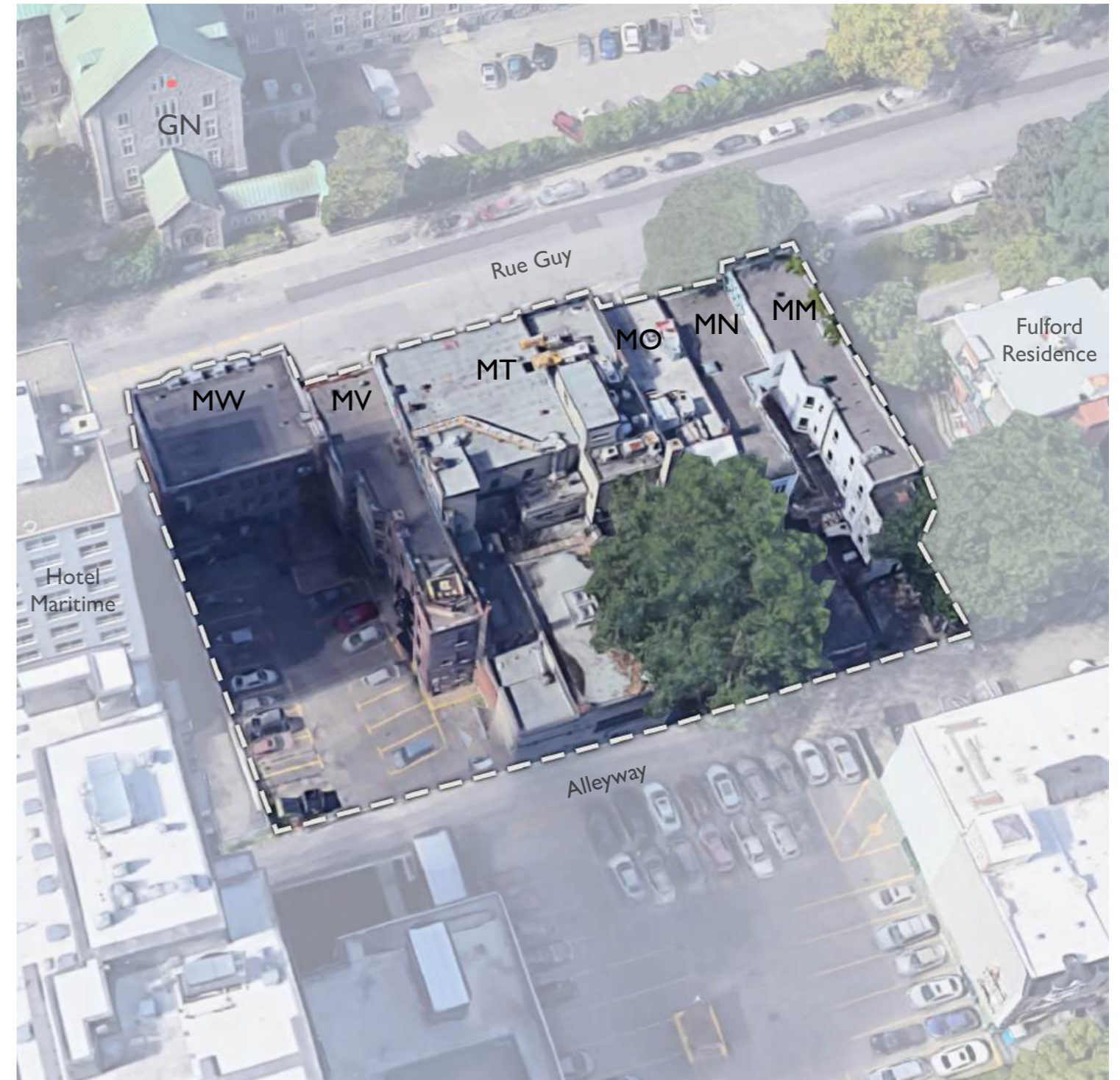
Aerial view of existing conditions
