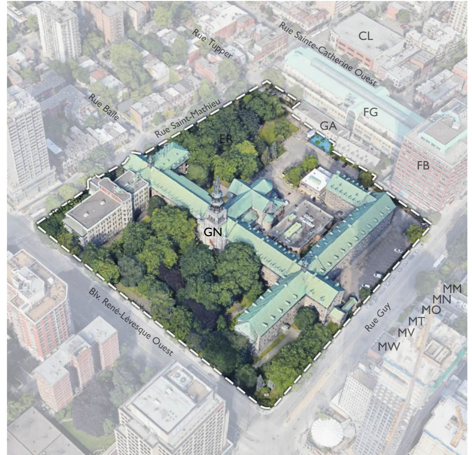
Aerial view of existing conditions
