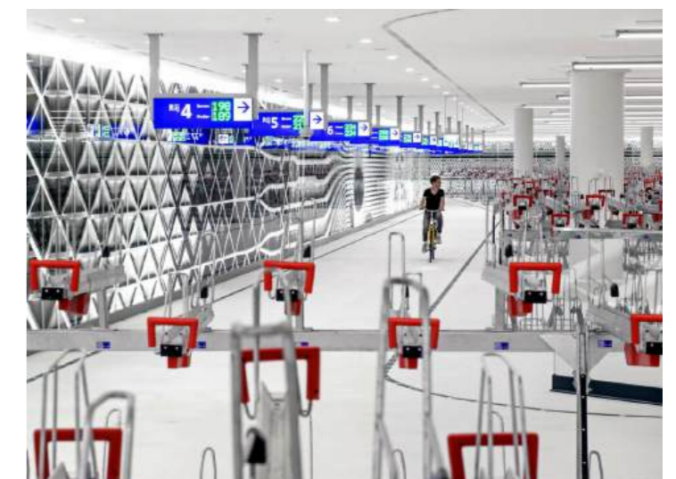
Indoor bike parking The Hague, Netherlands – Architect, SiloAgency, Mike Bink
