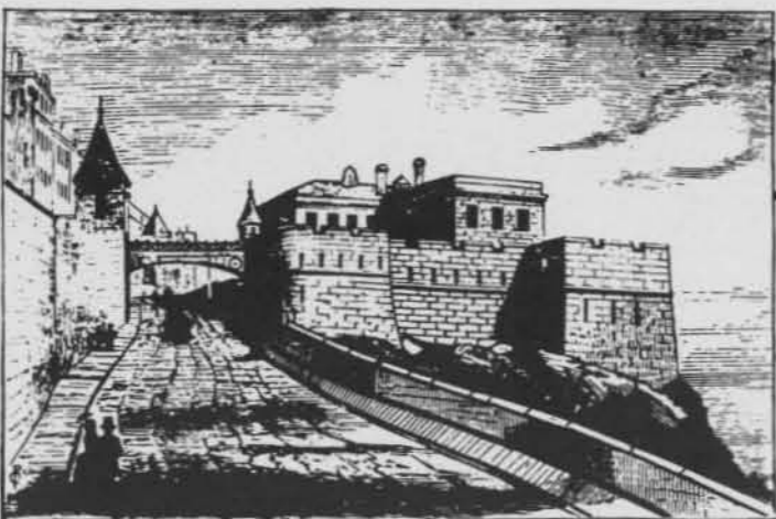
MOUNTAIN HILL.—Iron Bridge.
