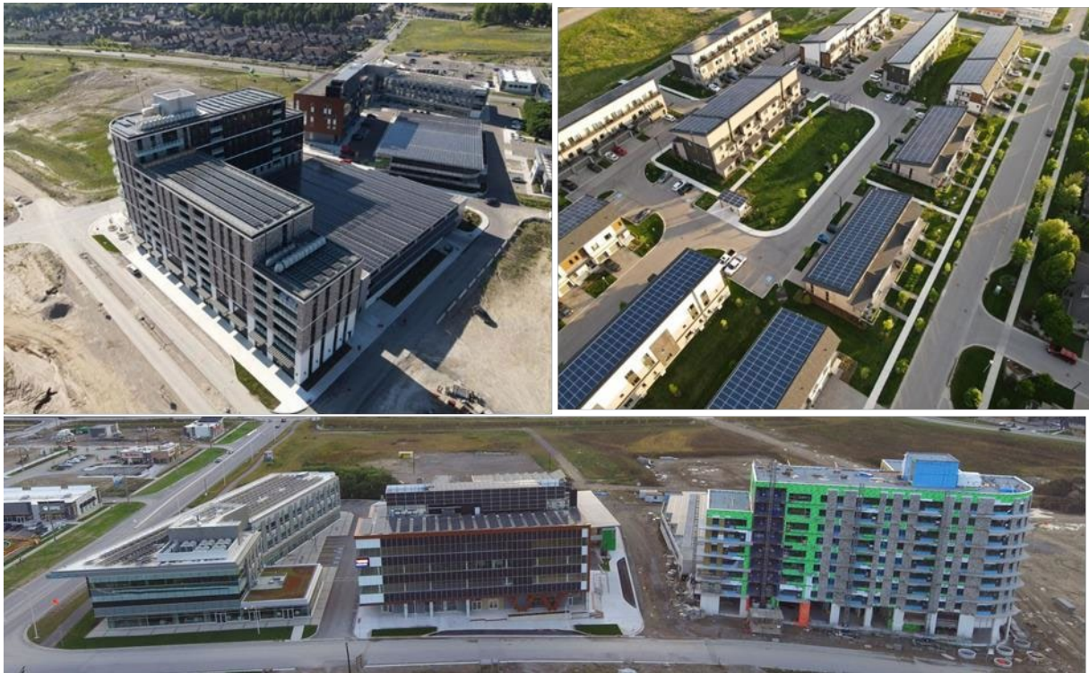
Figure 12: Various buildings in the West 5 community. 55
