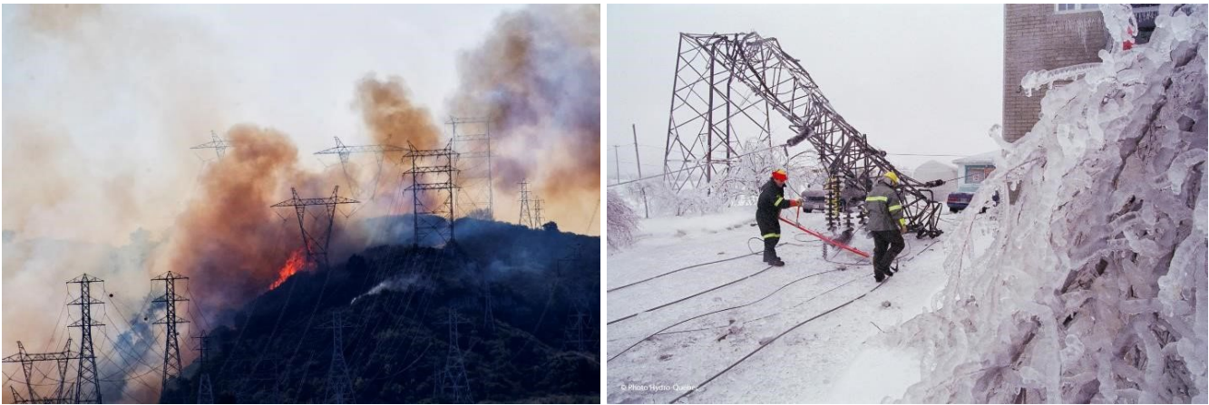
Figure 7: Experiences from forest fires 27 to ice storms 28 have shown how vulnerable electricity grids can be to extreme weather events. Building- and community-scale electricity generation and storage will be essential for making communities resilient to climatic shocks and extreme weather events.
