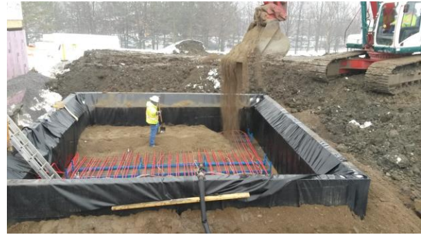
Figure 6. Sand based seasonal storage system.
